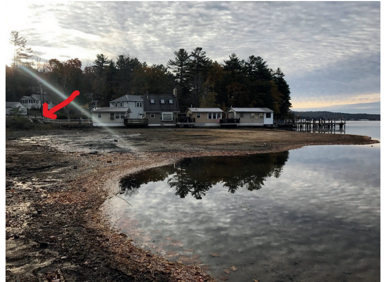
Langley Cove looking south toward Capri Condos. Red arrow marks the location where Langley Brook comes in under Weirs Blvd.
