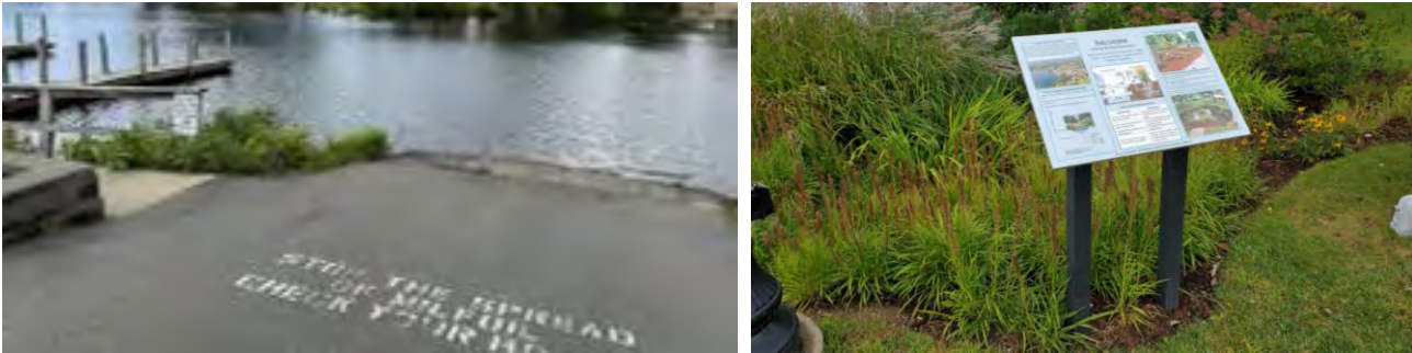
(Left) Runoff tends to move downhill rather than into the rain garden. A forebay would increase the amount of stormwater reaching the rain garden. (Right) Rain garden in Bean Park that could receive and treat runoff from the parking lot.
