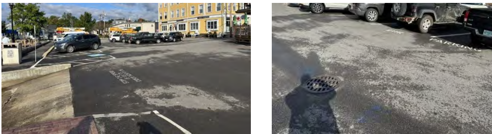
(Left) Large paved area between commercial buildings and the boat ramp. (Right) One of the drain inlets within the parking lot.
