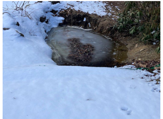
Caption: Makeshift infiltration trench on Sandy Cove Rd.
