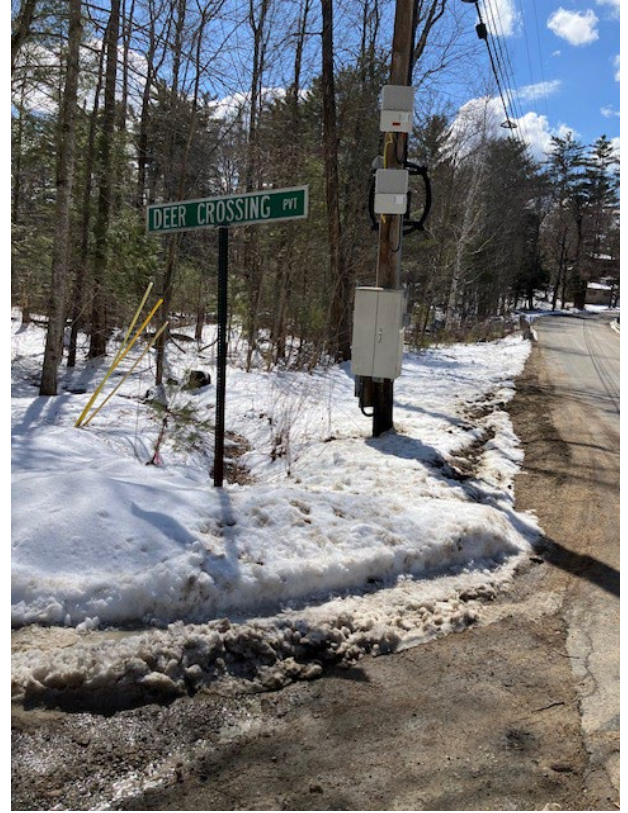
Runoff from roadway behind street sign flowing toward stream.
